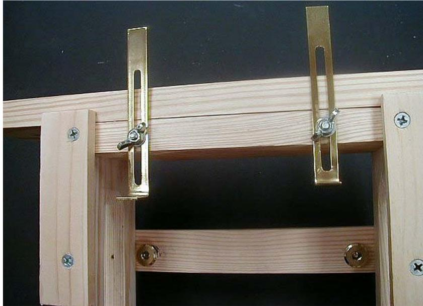
**Cut two strips 4  $\frac{3}{4}$  inches long. Insert each strip into a vise leaving a little more than  $\frac{3}{4}$  inches exposed. Bend that portion to form a 90 degree angle.**
